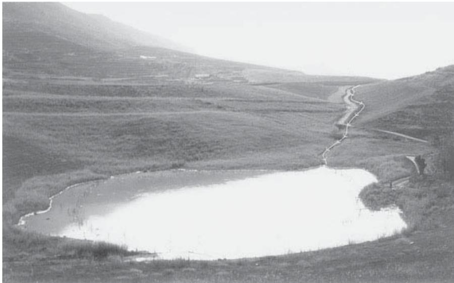
Figure 4. Constructed hydrological basin on a steep original relief. Artificial slopes still follow the platform-bank model. Reservoir works as a firebreaks line avoiding sediment emission to the natural watercourses and reducing peakflows.
