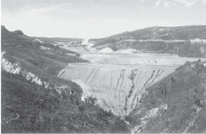
Figure 2. Filled-valley following the platform-bank model.
